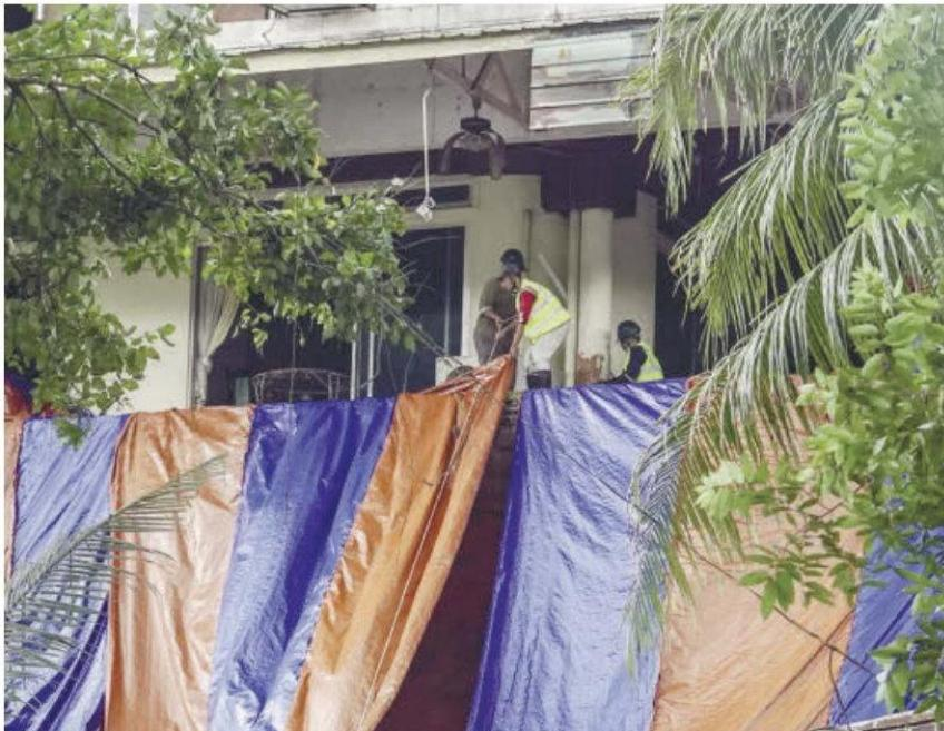
Tarpaulin sheets are used to cover the exposed slope following a landslide at Jalan Kemensah Heights.
